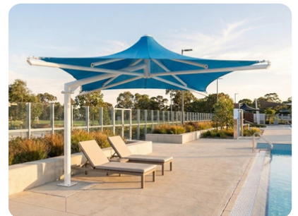
Aquatic centres UV cover for pools and decks | CANTILEVER
